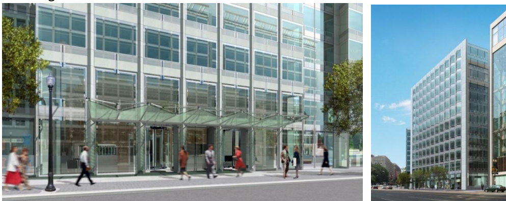
Figure 2 Main Lobby Entrance facing K Street (left) and perspective of curtain wall system (right)
