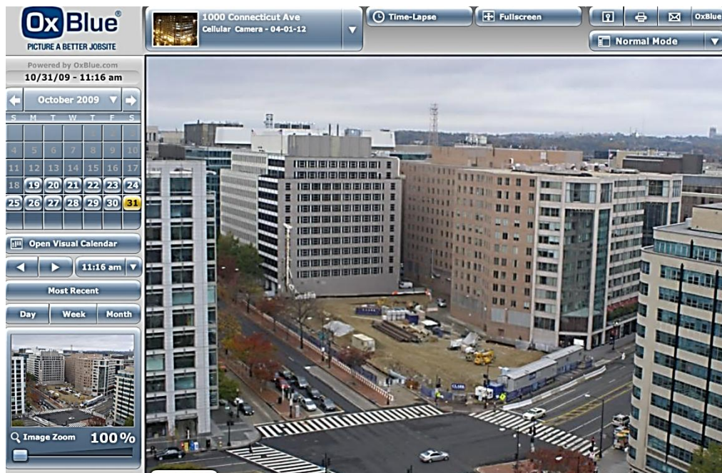
Figure 56 construction site before excavation (October 2009)
